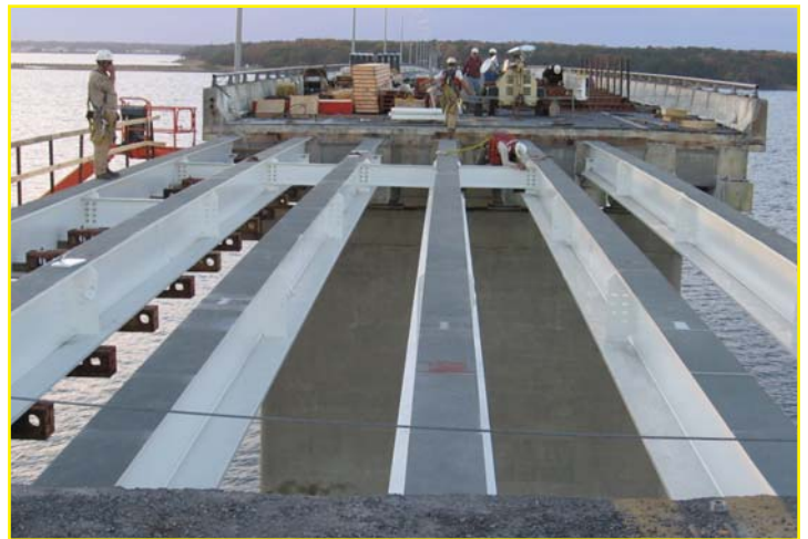
The Route 90 Bridge showing the erected steel
