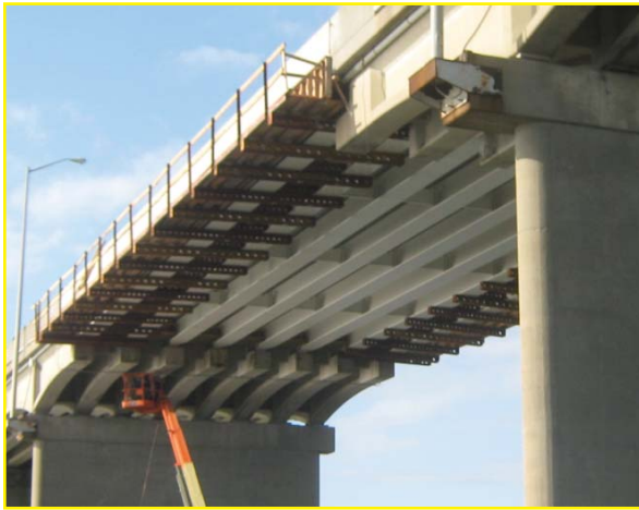
Finishing touches are placed on the new Route 90 Bridge navigational span
