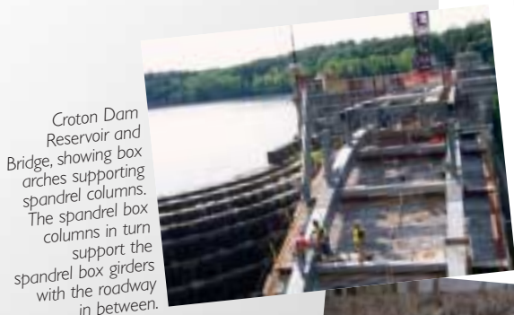
South abutment of Croton Dam Bridge showing the old structure supporting the fall protection and the new box arches without the keystone erected.
