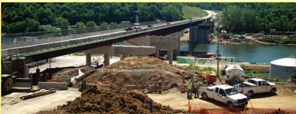
The Masontown Bridge under construction.
