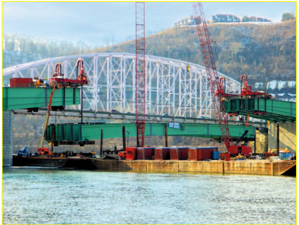
The final span of girders for the Hulton Bridge is strand-jacked into place
