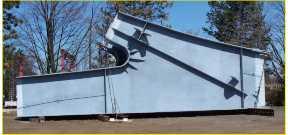
Metalized knuckle girder for the Lake Champlain Bridge.
