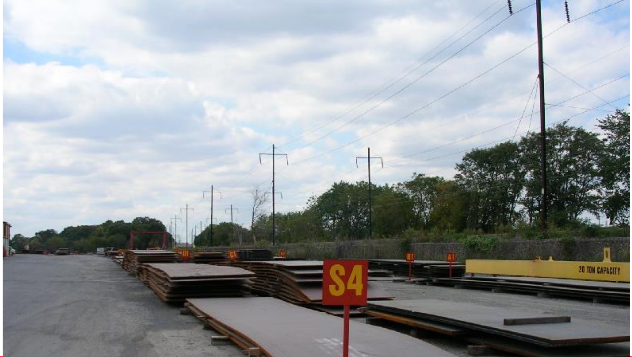
Fabrication – Stacking of plates
