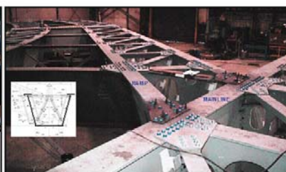
FIGURE B Merging Tub girders Curved & Skewed Geometry, Ramp Station Line Terminal
