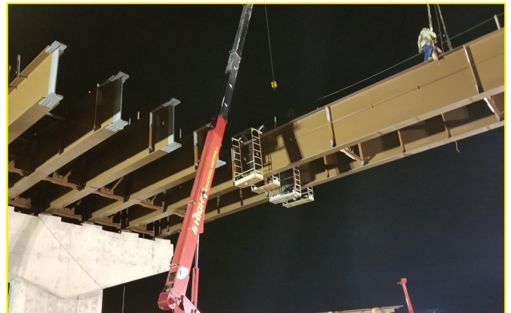
D10 PKF/HSE beam setting operations over PA Turnpike
