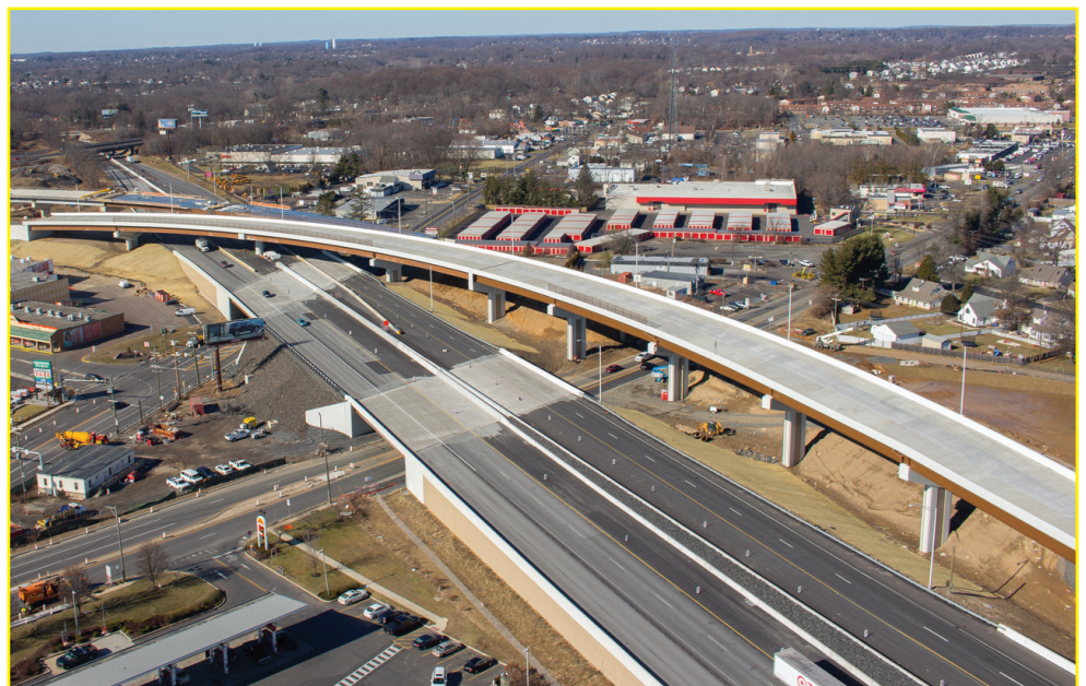
D10 Flyover PA Turnpike section
