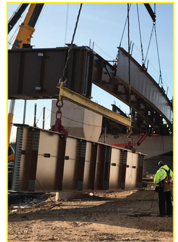
D20 section Nyleve/High Structural Erectors setting beams
