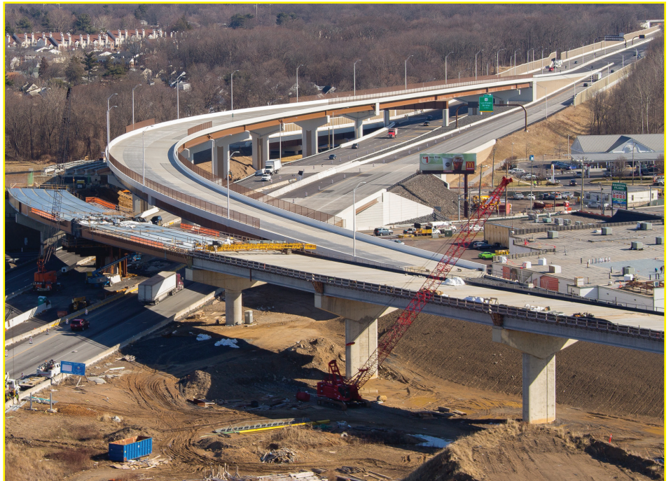
The long awaited I-95 and I-276 connection is open to traffic.
