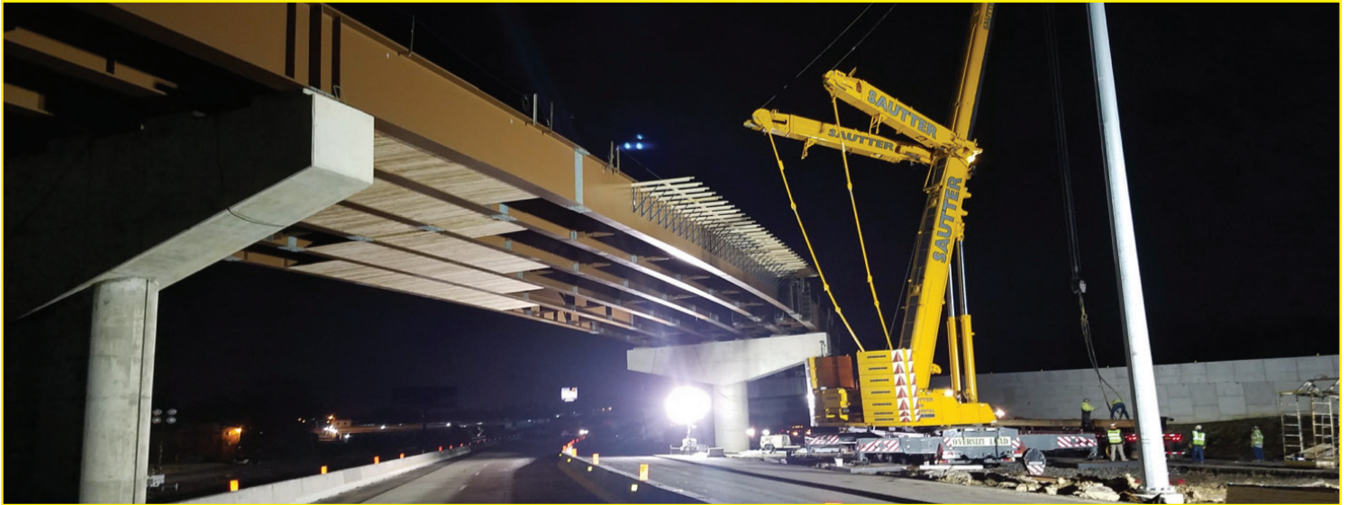
D10 PKF/HSE beam setting operations over PA Turnpike
