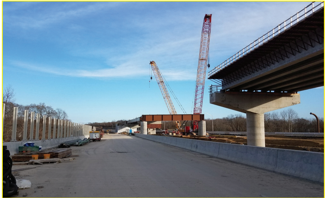
D10 section pier bent
