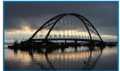
completed in two and a half hours. Crews hooked the arch onto four massive jacks and the arch was raised into place.
