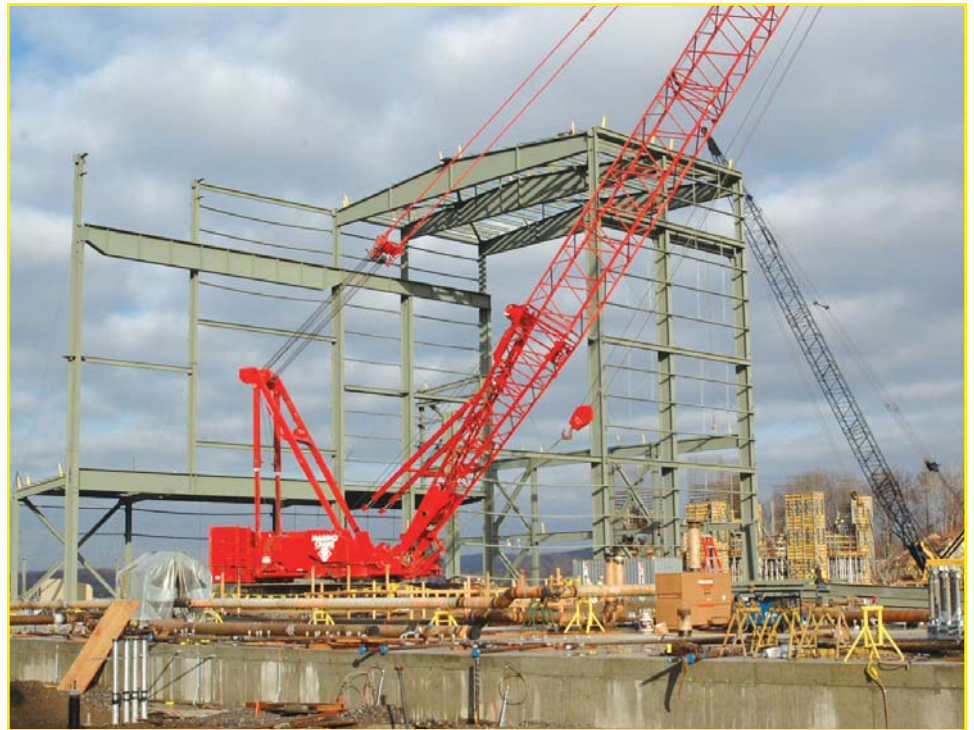
Kleen Energy plant under construction
