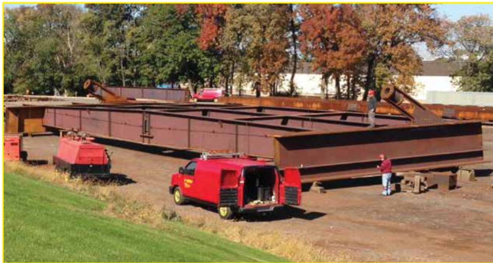
Grillage unit assembly in High Steel yard
