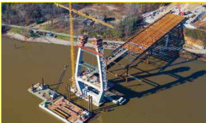
Backspan steel erection on falsework
