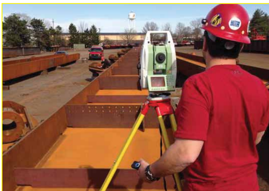
Typical Edge girder yard assembly measurement (anchor-to-anchor and field splice alignment)
