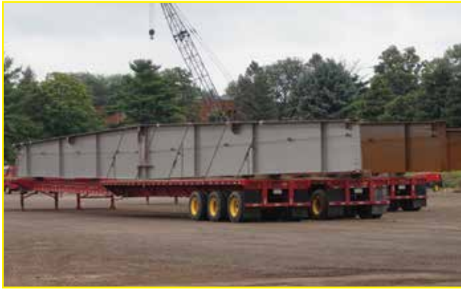
Floor beams loaded on trailer
