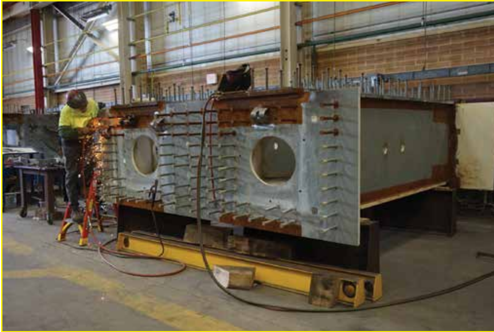
Tower anchor box in fabrication
