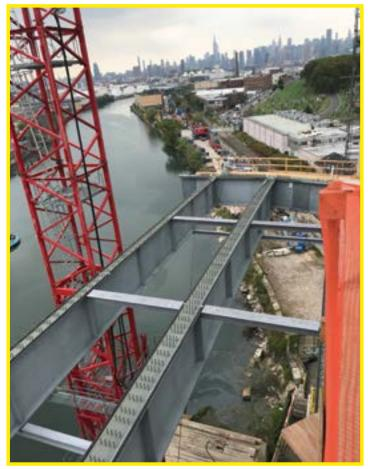
The bridges' metalized coating was chosen to reduce maintenance costs over a 100-year service life. Photo courtesy of Granite Construction Northeast
