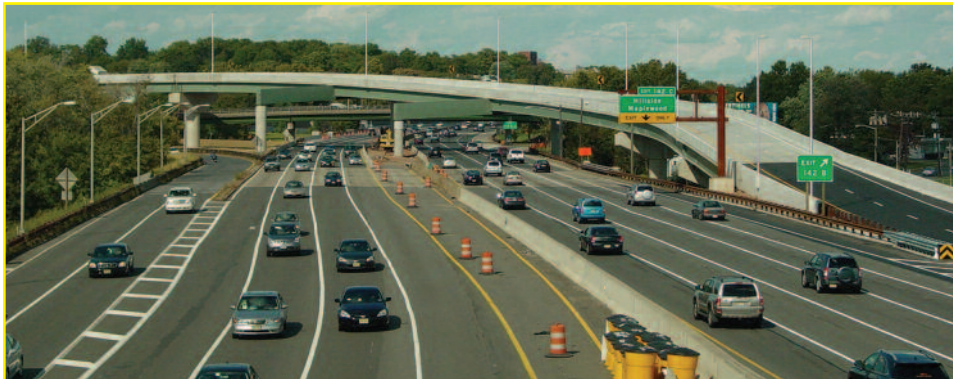
A view of Ramp NW-D at Interchange 142 of the Garden State Parkway.
