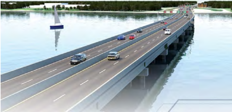
Low-Level Approach Spans
