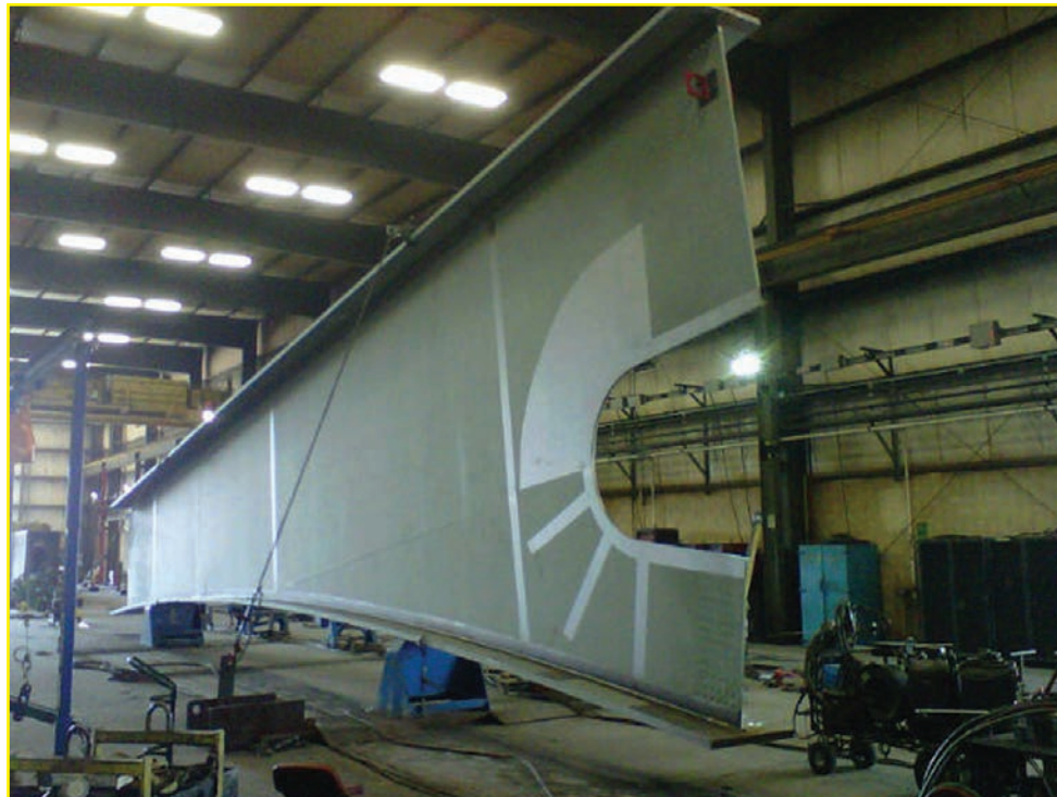
Knuckle girder in fabrication
