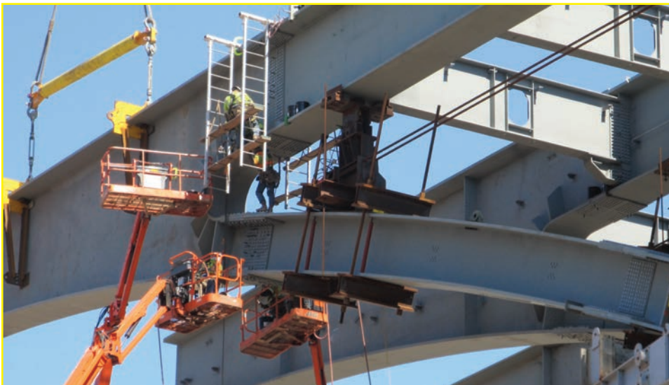
Erecting a Delta Frame - Courtesy Walsh/HNTB Innerbelt Project Team
