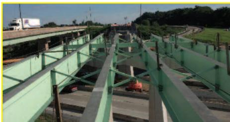
Usually, the structural steel is critical to getting the damaged bridge back in service, so owners look to the steel fabricator to fabricate and deliver the steel in the shortest time possible. When High Steel becomes a part of an Emergency Project all the stops are pulled out.
