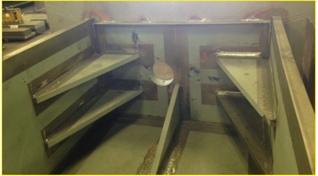
Figure 4 – Photo of five of the six internal bearing stiffeners at one end of one of the arch ribs.
