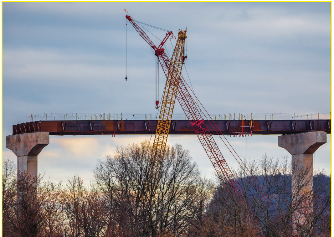
The first of 408 girders have been erected for the CSVT River Bridge. The girders are 10 feet tall, weigh 20 to 47 tons, and range from 74 to 122 feet in length.
