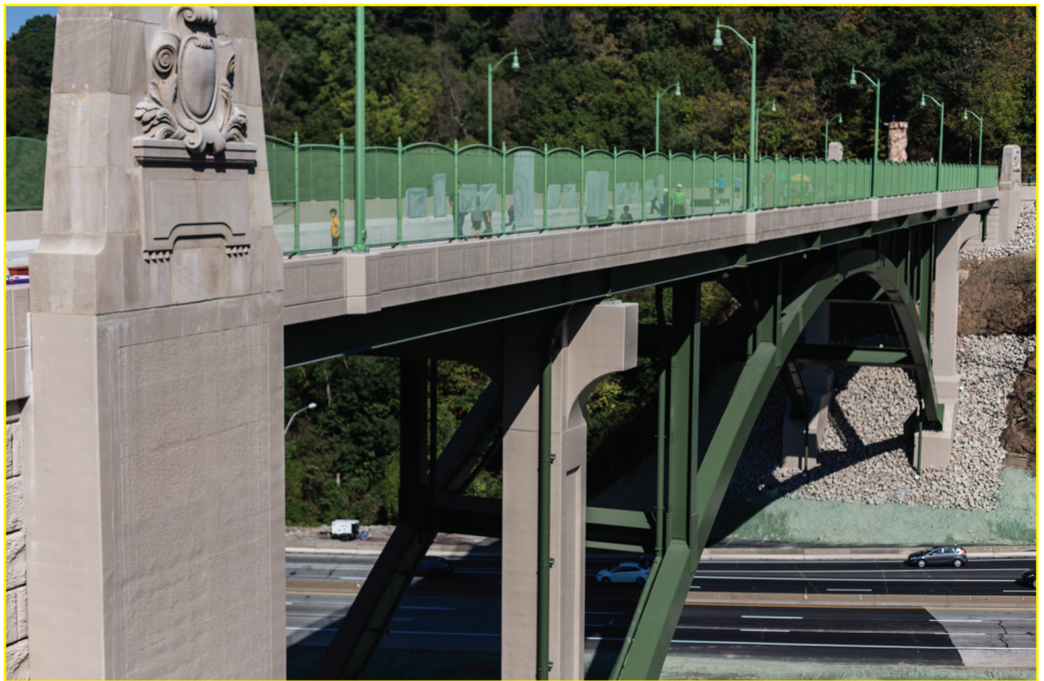
The Greenfield Bridge Project looking North
