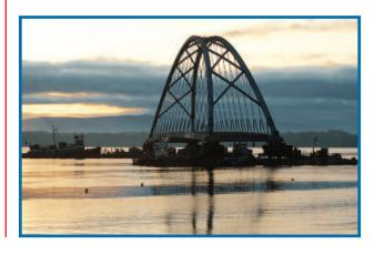
modified design allowed for enhanced redundancy, efficient use of steel, a replaceable deck, a lighter weight superstructure and reduced construction costs.
