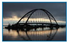
completed in two and a half hours. Crews hooked the arch onto four massive jacks and the arch was raised into place.
