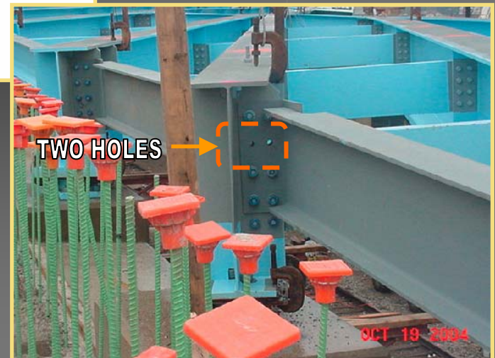
Minor, localized mis-alignment
