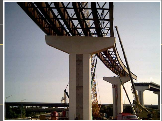
I-95 SB Ramp over I-95/I-395/I-495 Fairfax County, VA Fabricator, Erector: High Steel Structures Inc.
