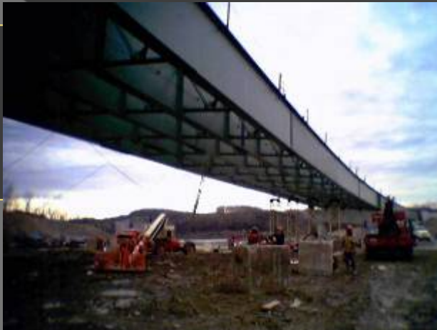
A) LATERAL STAYS (SHOWN HERE STABILIZING PRE-BD 620M TYPE PA STRUCTURE, CENTRE COUNTY PA)
