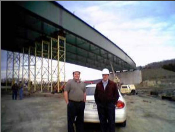
B) SHORING TOWER FOR VERTICAL LOAD/DEFLECTION CONTROL (SIMILAR TO ABOVE CENTRE COUNTY, PA STRUCTURE TO LEFT OF DISTINGUISHED GENTLEMEN)
