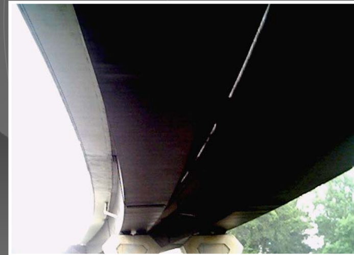
WMATA Blue Line over I-95 Prince George's County, MD Fabricator, Erector: High Steel Structures Inc.
