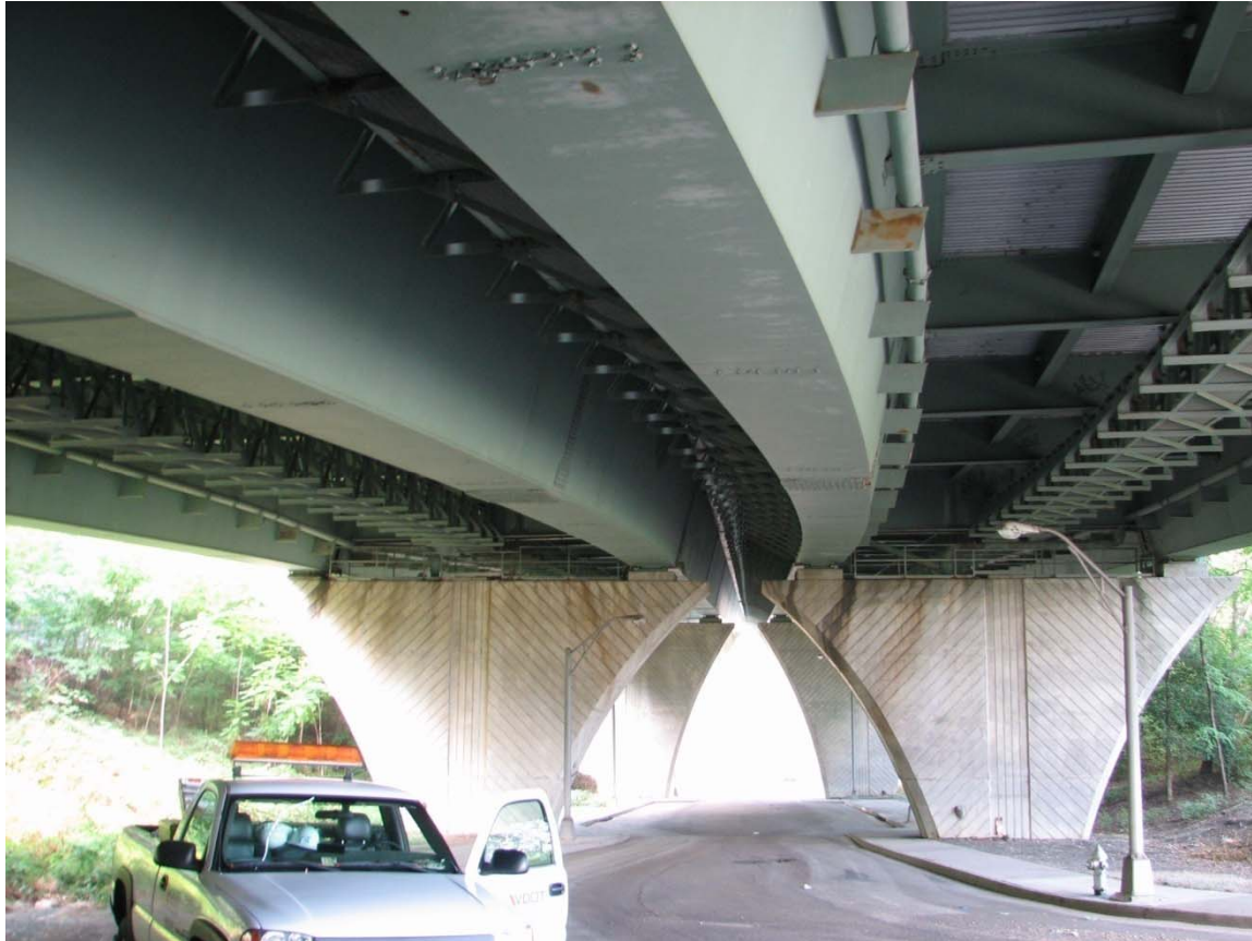
Martin Luther King Bridge 006
