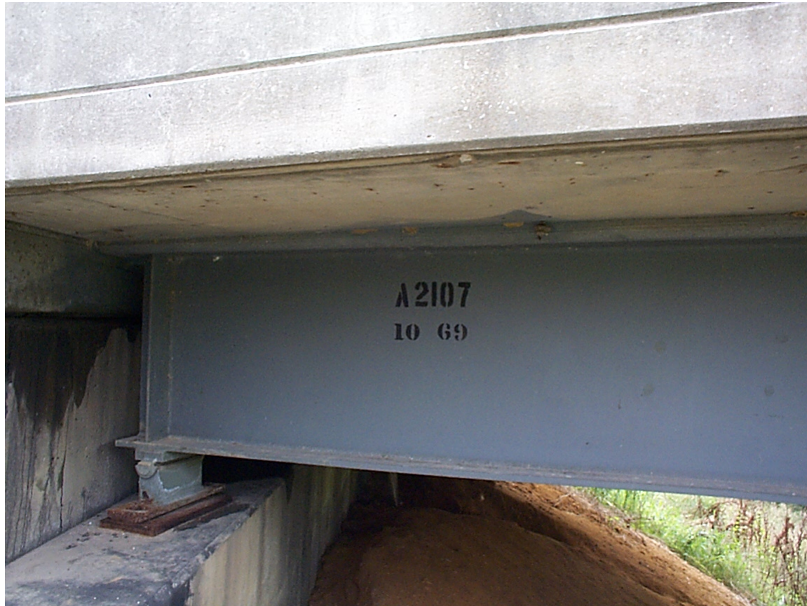
MoDOT Bridge No. A2107 over Pin Oak Creek after 30 years (1999).
