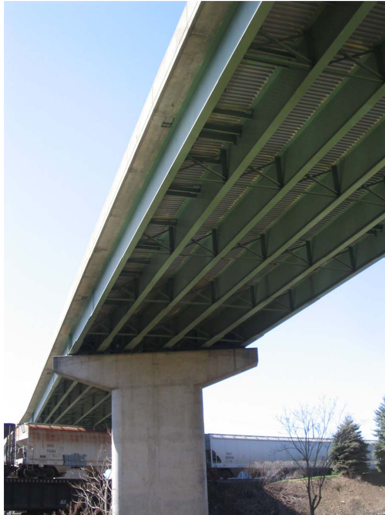
Windgap Bridge – General view of bridge showing typical good condition of coatings
