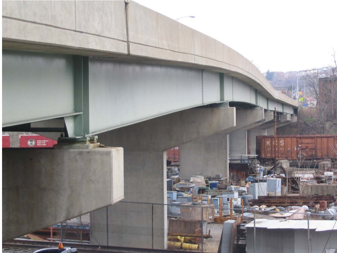
Windgap Bridge – Typical good coating appearance on various bridge members
