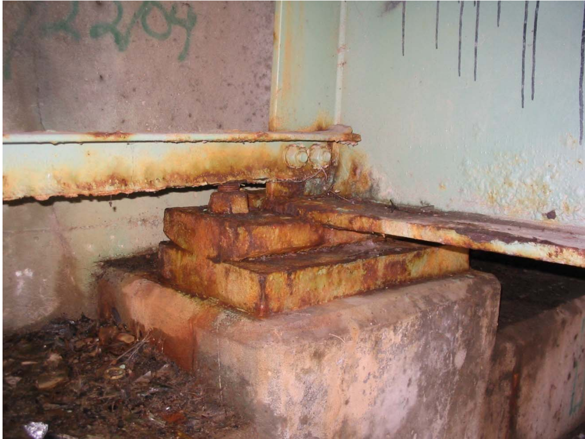
Windgap Bridge – Isolated rusting and coating breakdown at bearing/girder/end-frame connection beneath leaking north abutment expansion joint
