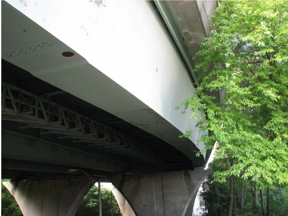
Martin Luther King Bridge 005
