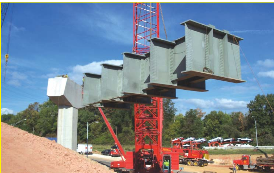
The same pier cap is erected using a 300-ton Manitowoc Crawler crane.
