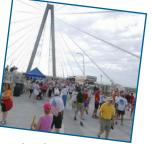
the largest single project in our history. It is indeed a modern marvel, at 3.5 miles and eight lanes. The huge bridge was constructed with more than 24,000 tons of fabricated steel and a main span that is the longest cable-stay in North America at 1,750 feet.
