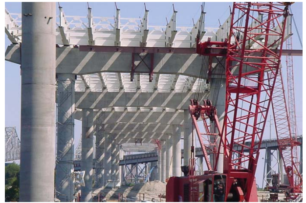
The new Cooper River Bridge is primed with inorganic zinc.
